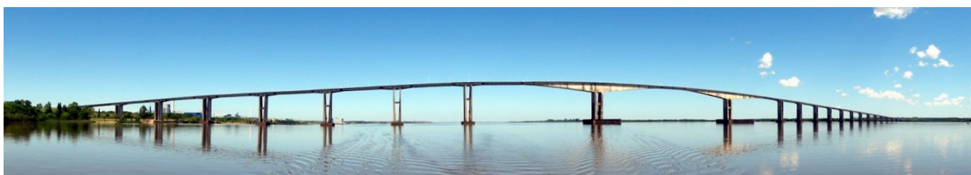
Libertador General San Martín Bridge looking east This is a cantilever road bridge that crosses the Rio Uruguay and joins Argentina and Uruguay
