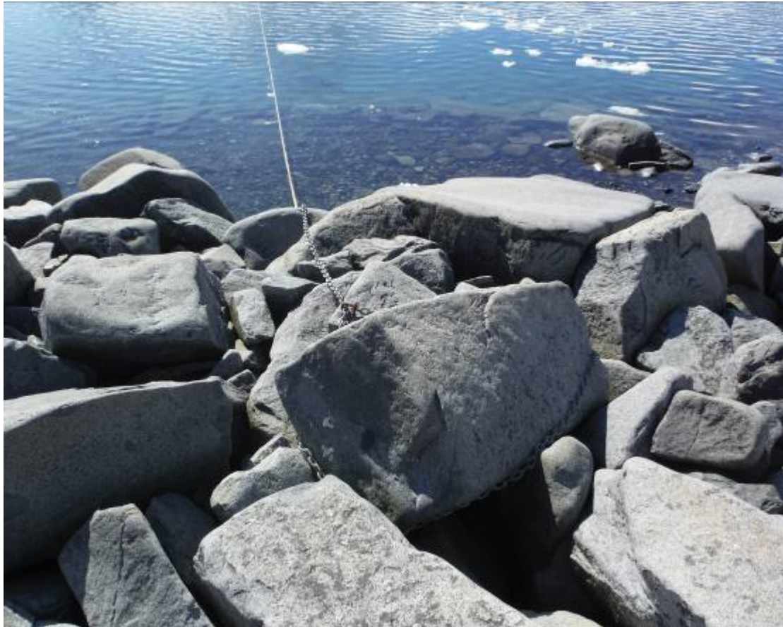
Wiencke 8 Mooring line attached to a chain sling around a large boulder.
